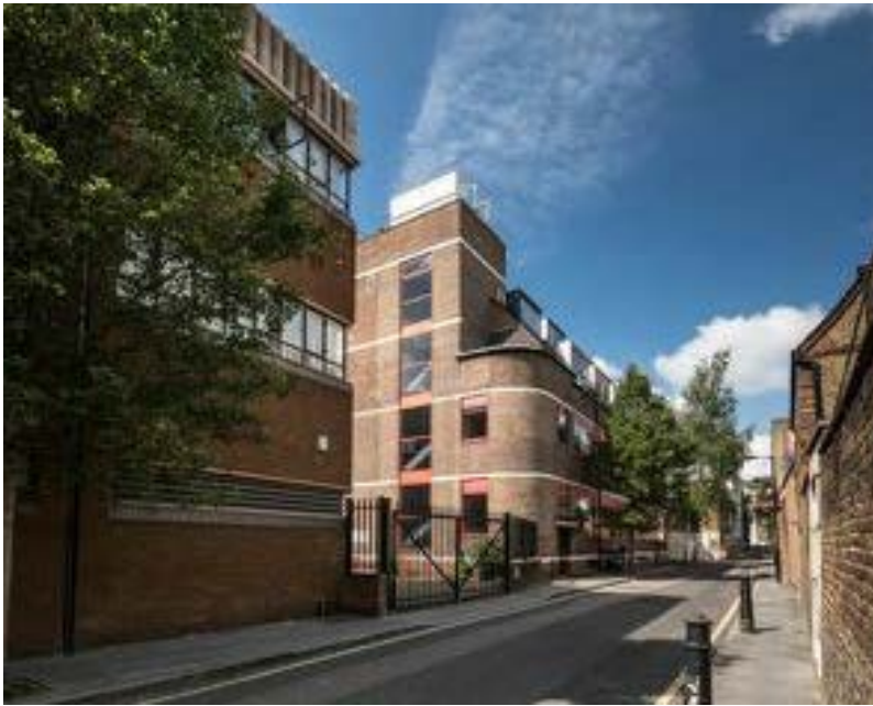
View from Copperfield Street
